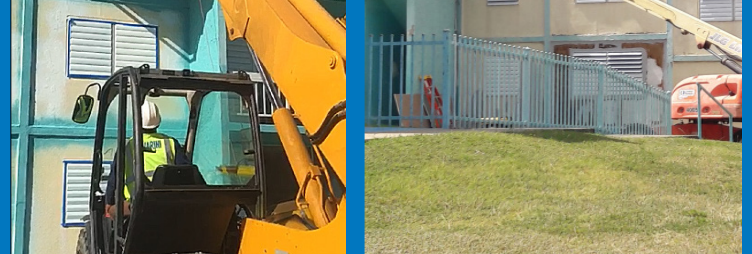
Installation of elevator.
